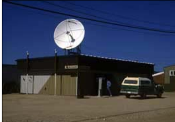
Satellite and Internet communications have helped to open up the North
